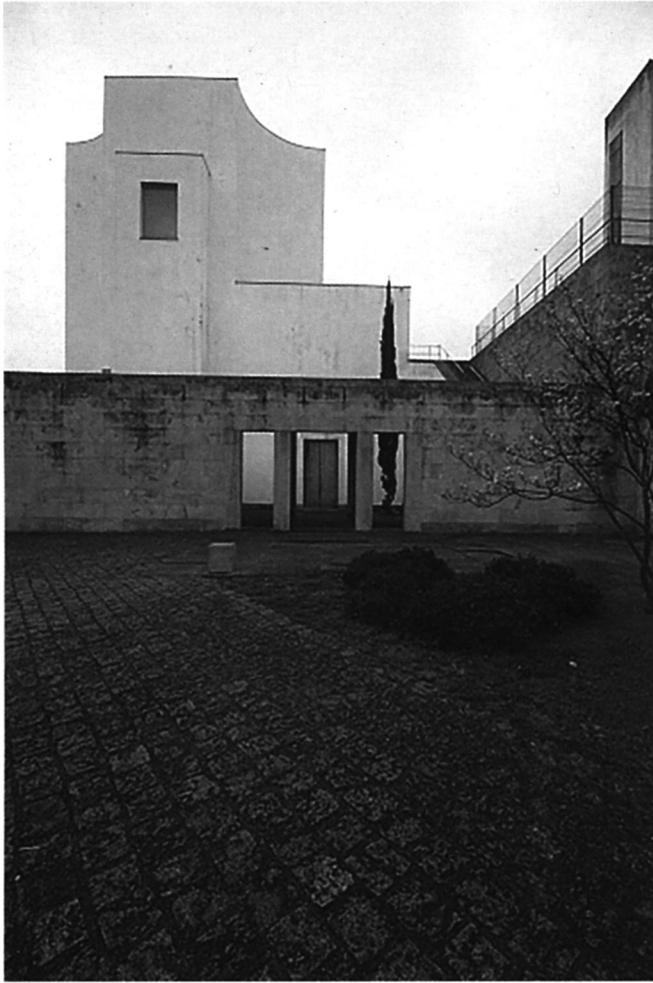
View from the garden looking west towards the crypt.
